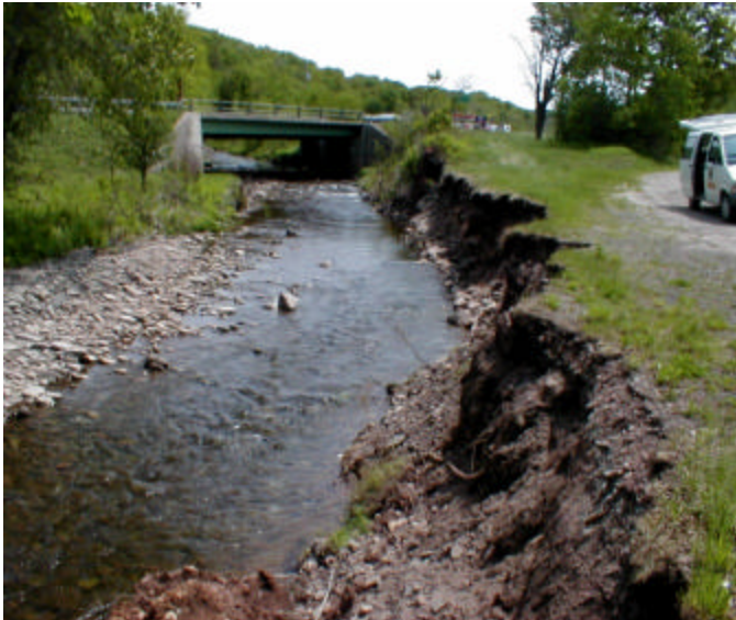
Problem Reach 1.1 Example of a rapidly eroding steep bank on a Rosgen B4 stream reach. Dominant substrate is coarse gravel.
