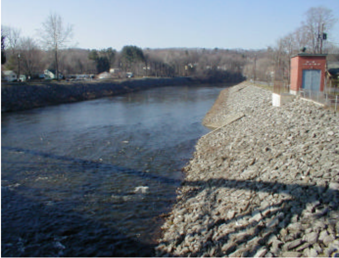
Problem Reach 3.5 Example of a channelized, leveed, rip rapped F3 stream reach
