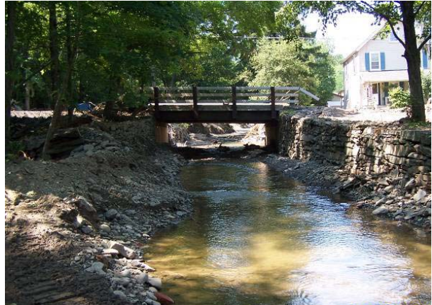
Figure 2.18 Bridge results in elimination of Floodplain
