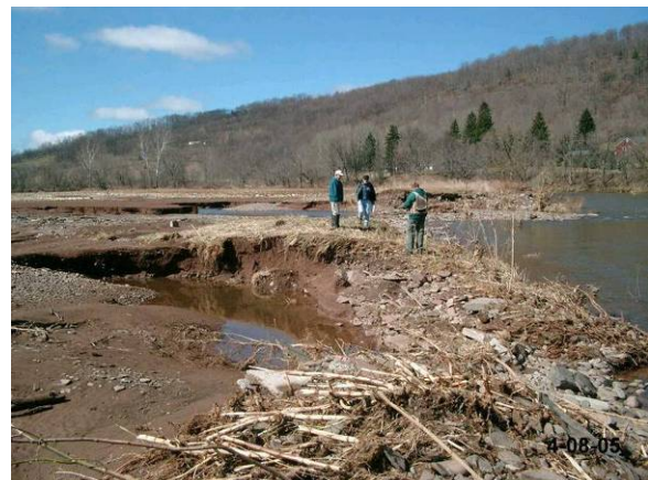
Figure 3.12 Berm that was breached in 2005 storm event
